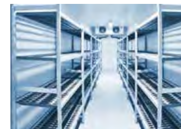
Solar Cold Storage Free Day Time Cooling
